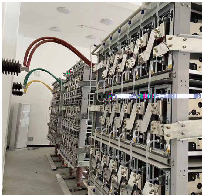
Water cooling system
