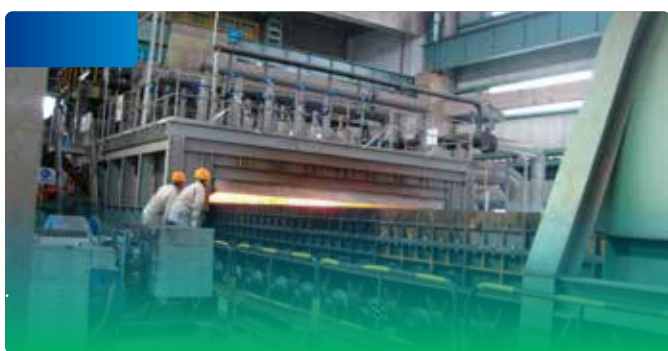
Metallurgy: main extractor fan, blast furnace blower, dust removal fan, slurry pump, descaling pump, centrifugal feed pump, elevator, semi-automatic mill, etc.
